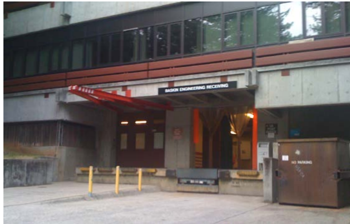
Figure 2. JBEB Loading Dock
